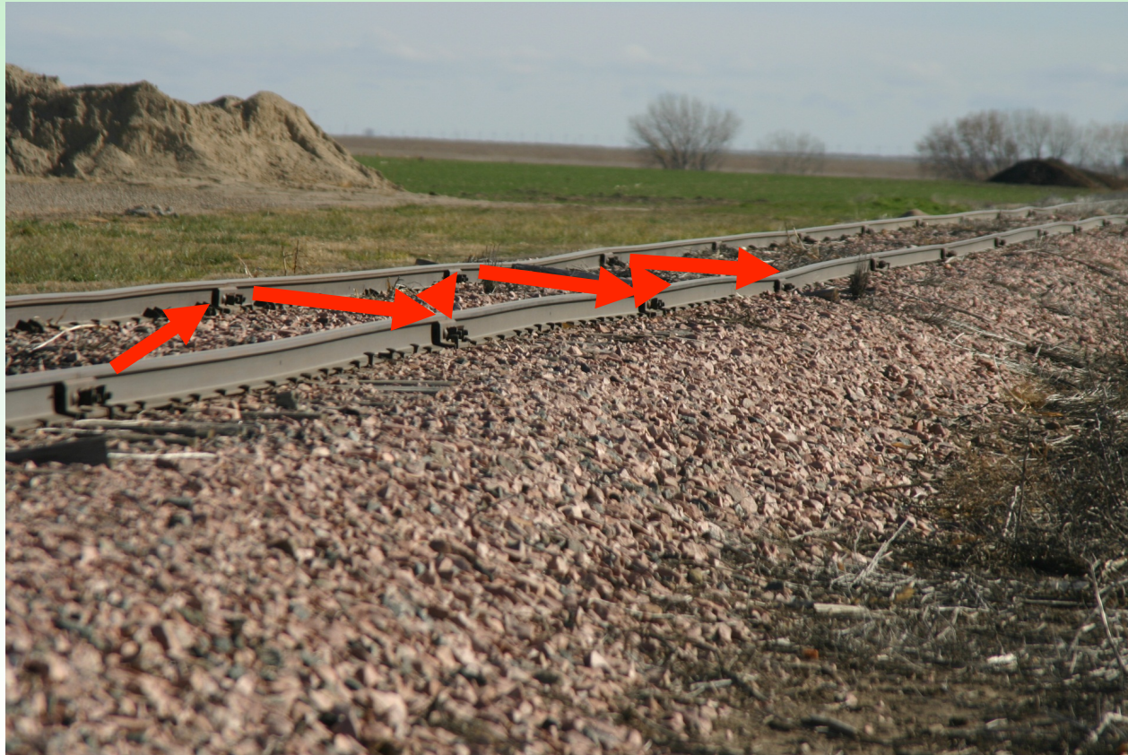
Staggered Jointed Rail
