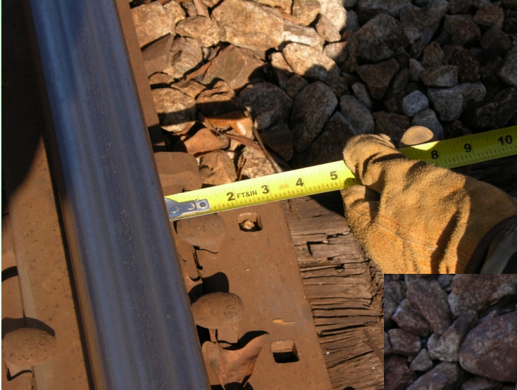
Measuring gage 5/8" below head of rail
