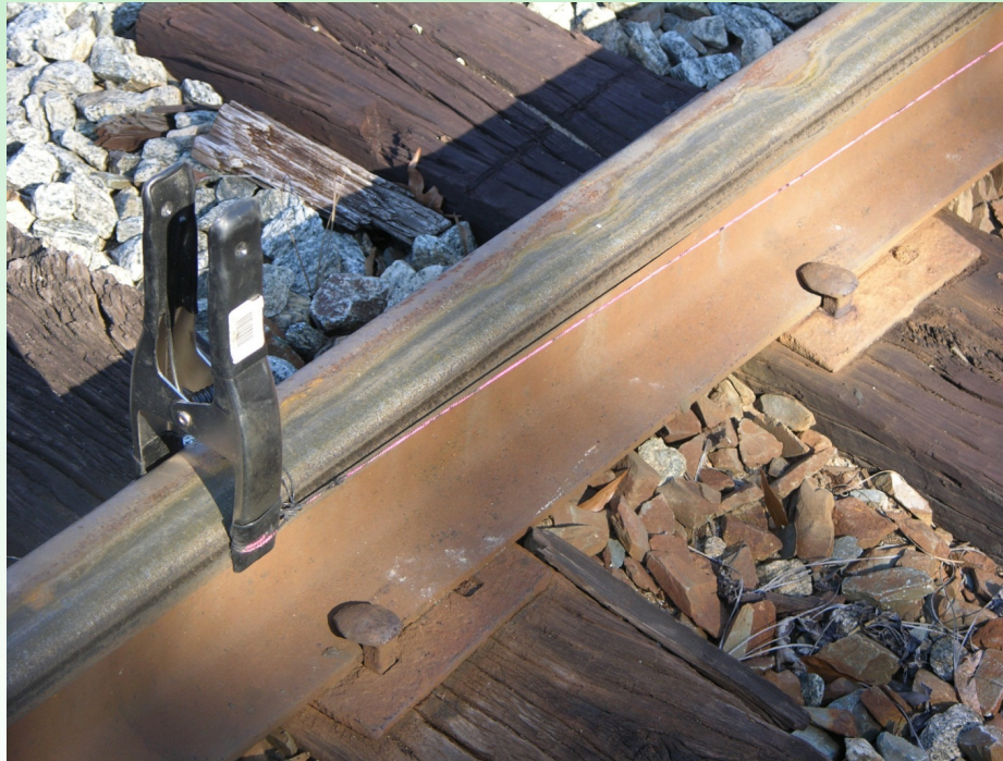
Using Spring clamps to Stringline when no help available
